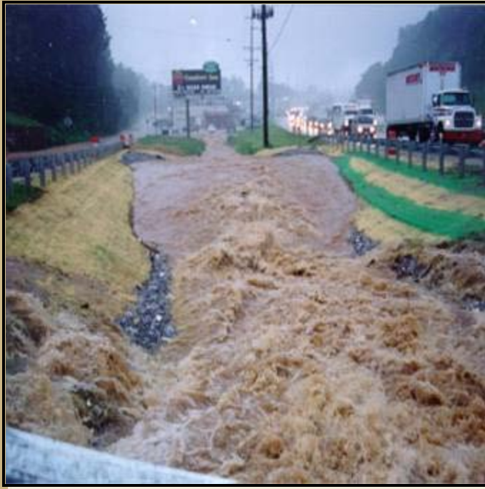
More Frequent Flooding
